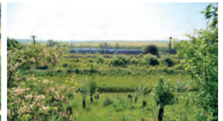
Earth bund offering sound protection from high speed train line Moissy-le-Neuf (in the east of the Paris region)
