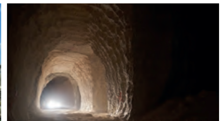
Backfilling of a gypsum mine Baillet-en-France (north west of The Paris region)
